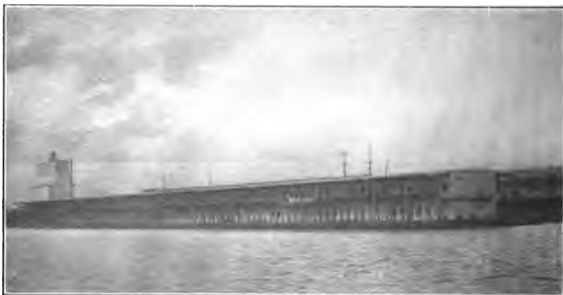
FIG. 89.—Water end view of Commandacia and Tarragona docks, Pensacola, Fla.— Louisville & Nashville.
