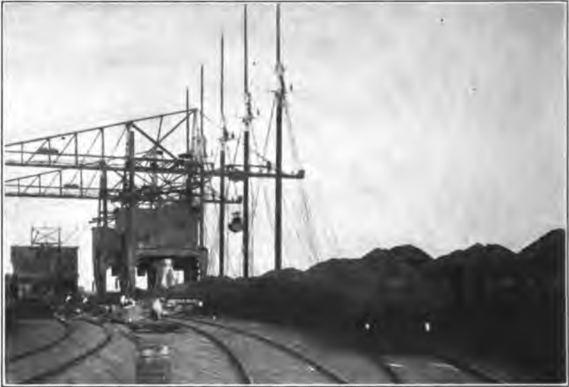
FIG. 99.—Coal discharging plant at Providence, R. I.—New York, New Haven & Hartford.
