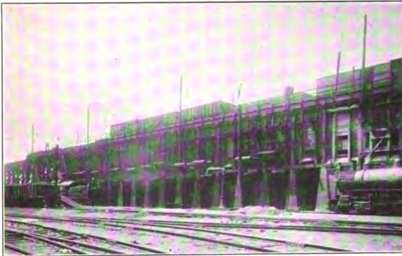
FIG. 200.—View of coaling plant, East Altoona—Pennsylvania Railroad.
