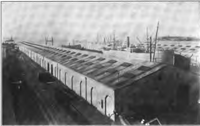
FIG. 80.—Covered pier of Bush Terminal.
