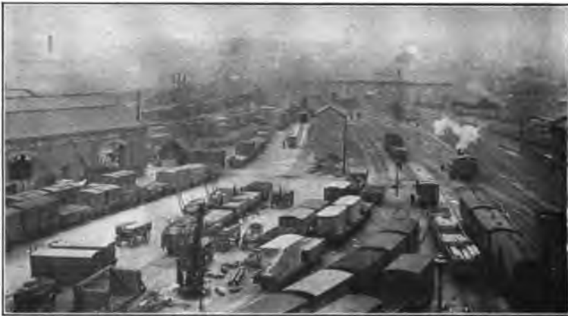
FIG. 143.—Camden goods station and yards—London & North Western.
