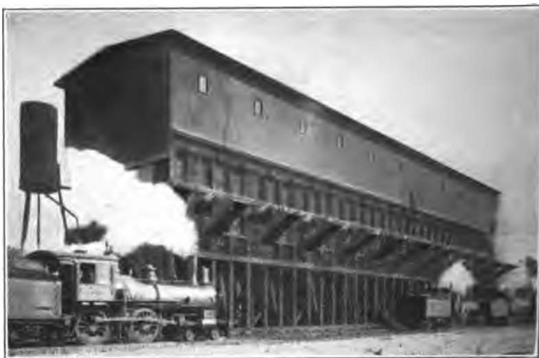
FIG. 195.—Coaling plant at Chicago—Chicago & North-Western.
