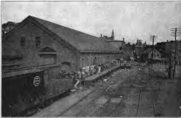
FIG. 120.—Inbound freight-house, Worcester, Mass.—New York, New Haven & Hartford.
