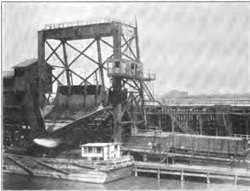
FIG. 98.—Car dumping machine, Hoboken, N. J.—Lackawanna.
