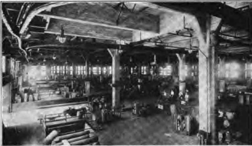
FIG. 154.—Interior of team floor, St. Louis Terminal—Missouri, Kansas & Texas.
