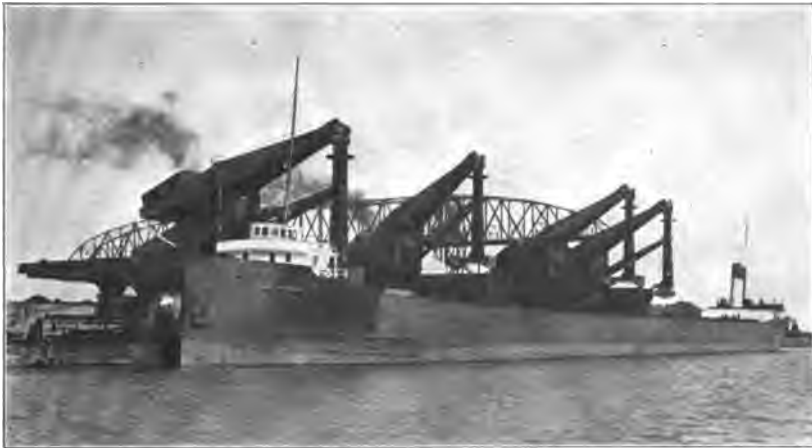
FIG. 106.—Mechanical (Hulett) unloaders at Buffalo.
