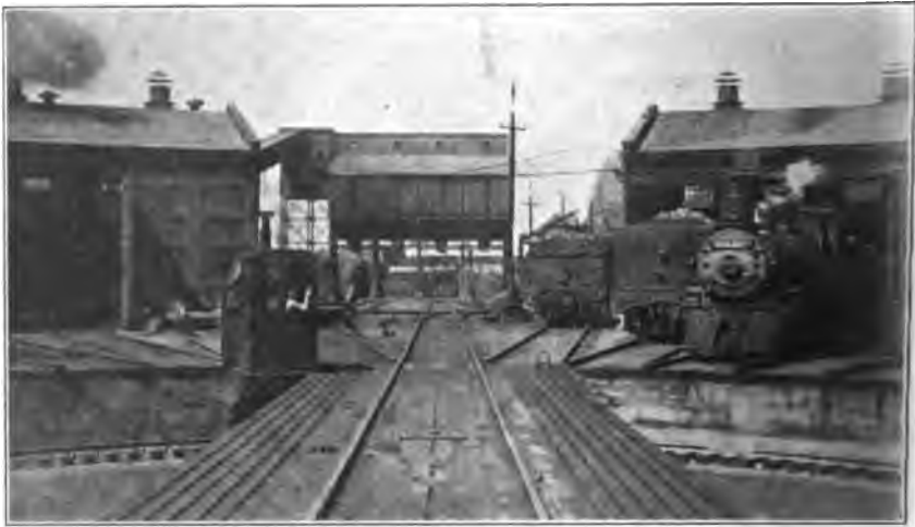
FIG. 177.—Engine-house, showing coaling-plant portion, Allegheny, Pa.—Pennsylvania Railroad.
