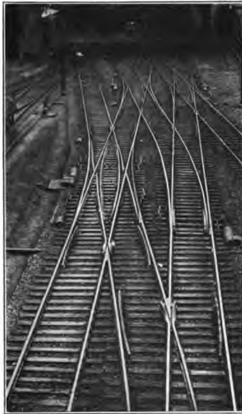
FIG. 17.—Typical easy-lead cross-overs.
