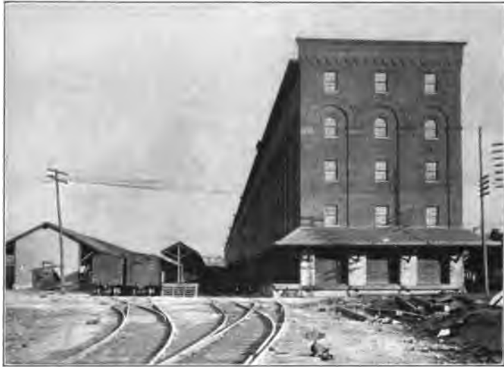
FIG. 123.—Track side of warehouse, showing transfer platform, Cincinnati—Baltimore & Ohio-Southwestern.
