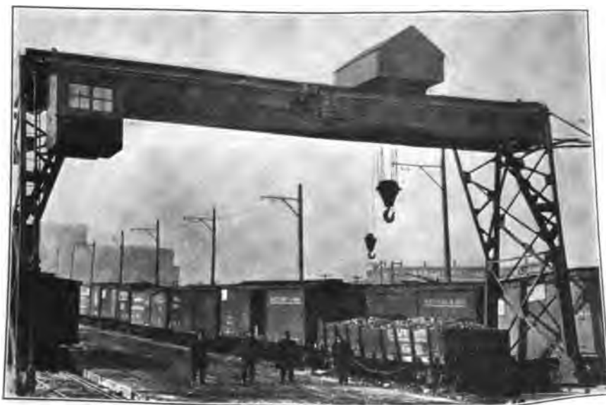
FIG. 52.—Electric power crane—Baltimore & Ohio.
