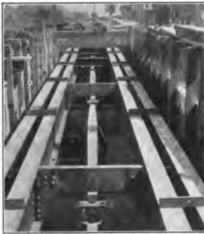
FIG. 66.—I-beams for bridge, track scale—Baltimore & Ohio.
