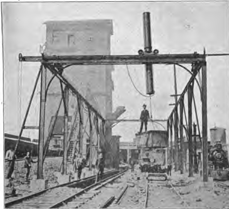
FIG. 207.—Pneumatic ash-handling plant for the Baltimore & Ohio.
