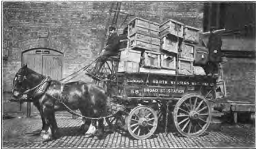
FIG. 139.—Freight dray, Broad Street Station—London & North Western.
