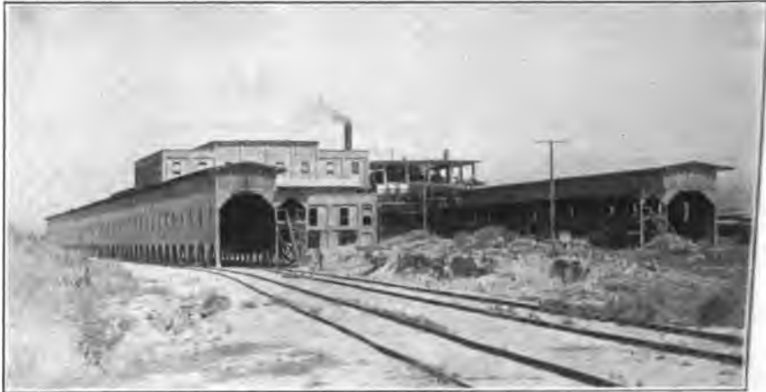
FIG. 166.—General view, pre-cooling plant, Roseville, Cal.—Southern Pacific.
