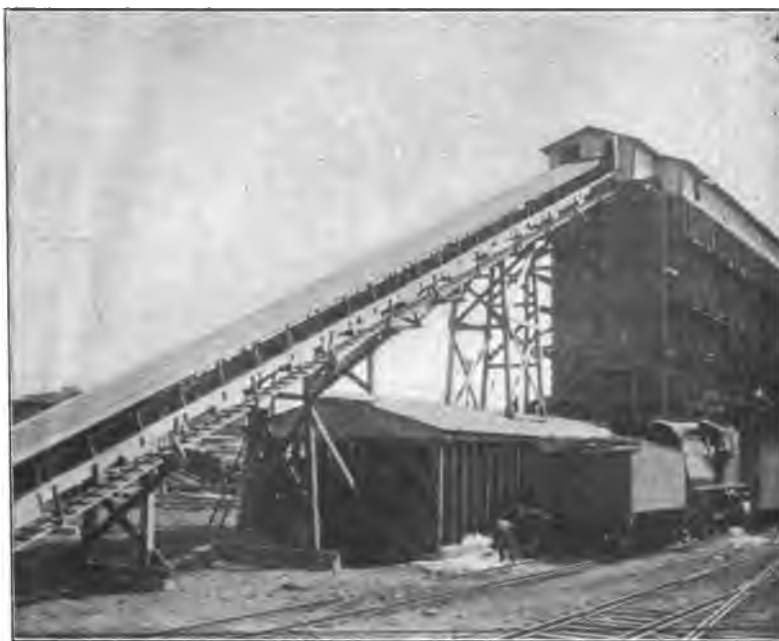
FIG. 197.—Conveyor Incline, Elizabethport coaling station—Central of New Jersey.
