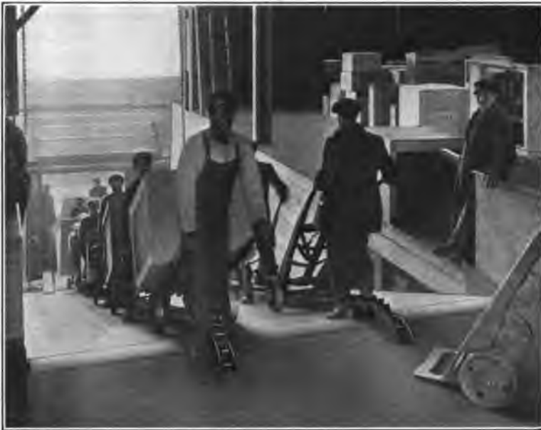
FIG. 159.—Inclined drop elevators, used by Merchant & Miner's Transportation Company.
