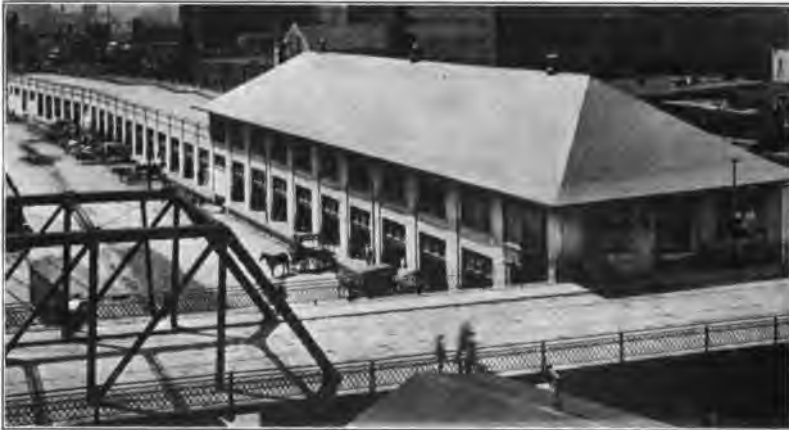
FIG. 115.—Inbound freight-house, Chicago—Baltimore & Ohio.
