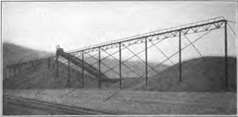
FIG. 102.—Coal storage plant, Ransom, Pa.—Lehigh Valley.
