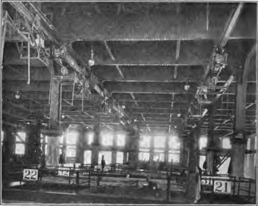
FIG. 153.—Telfers on runways above hatches, St. Louis Terminal—Missouri, Kansas & Texas.
