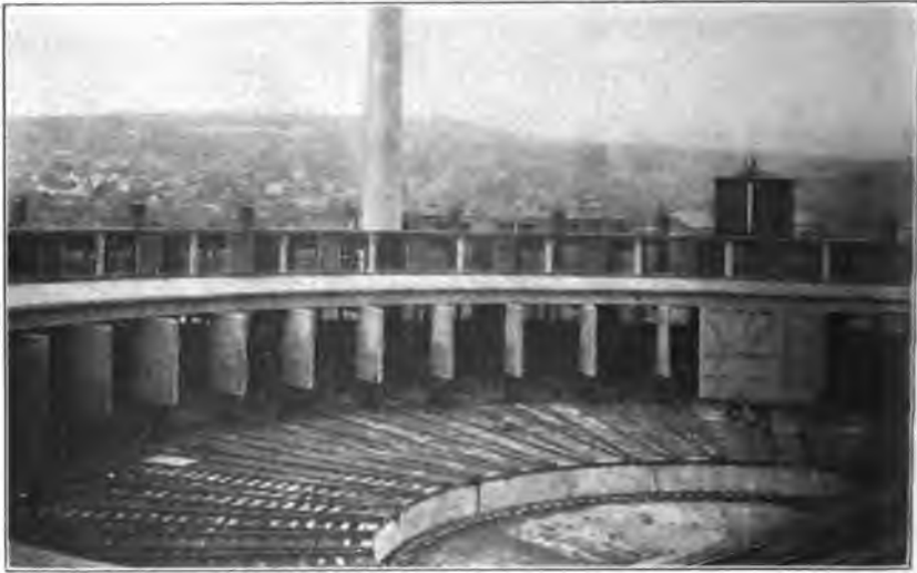
FIG. 189.—Inside circle view of Carbondale engine-house.
