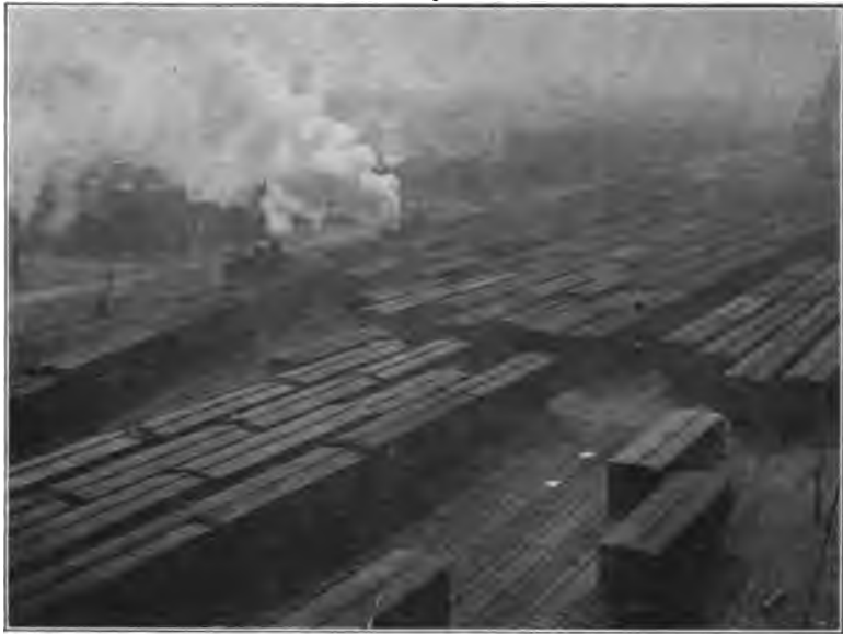
FIG. 84.—Yards of Bush Terminal.
