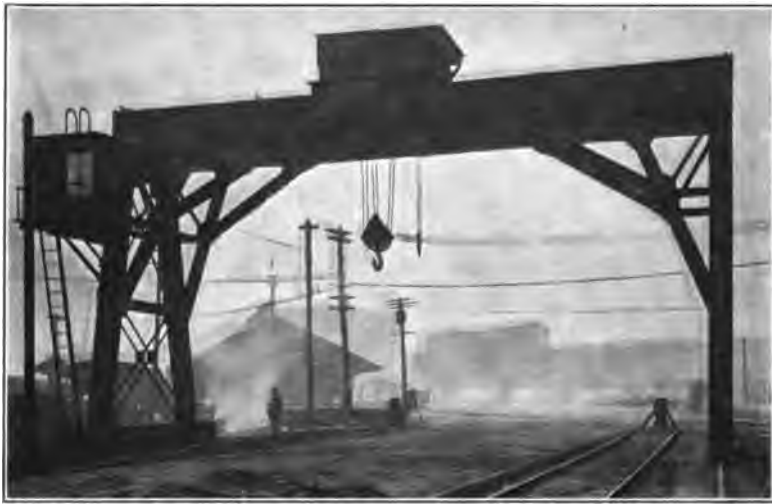
FIG. 51.—Typical freight transfer crane.
