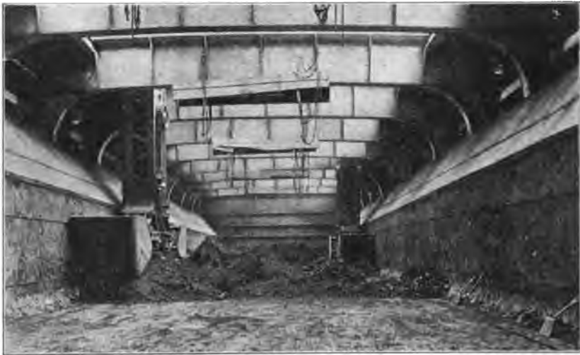
FIG. 107.—Leg of Hulett unloader in boat.
