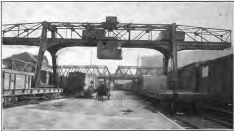
FIG. 53.—Electric traveling crane, Chicago—Lake Shore & Michigan Southern.
