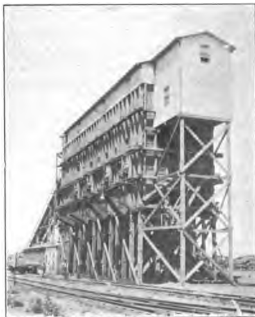
FIG. 196.—Coaling plant at Elizabethport, N. J.—Central of New Jersey.
