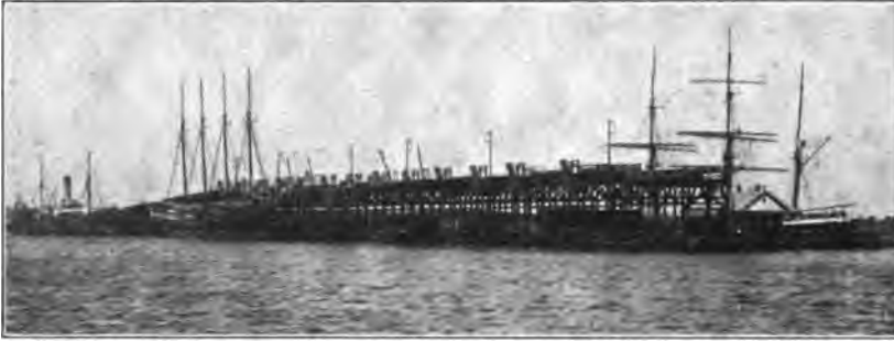
FIG. 86.—Coal, grain and lumber dock, Pensacola, Fla.—Louisville & Nashville.
