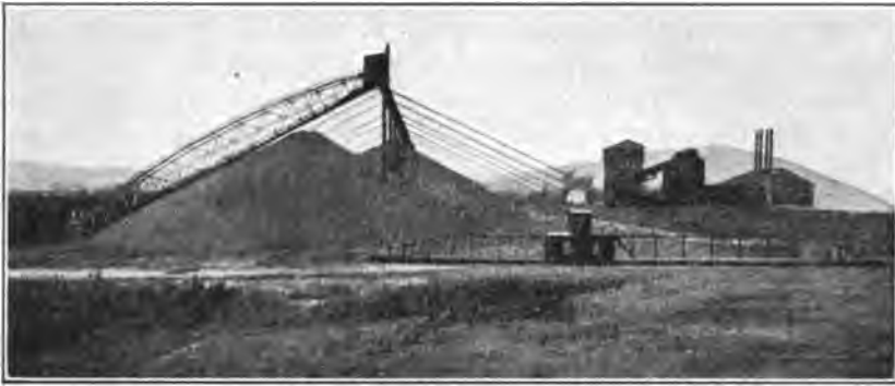
FIG. 103.—Coal storage plant, Ransom, Pa.—Lehigh Valley.
