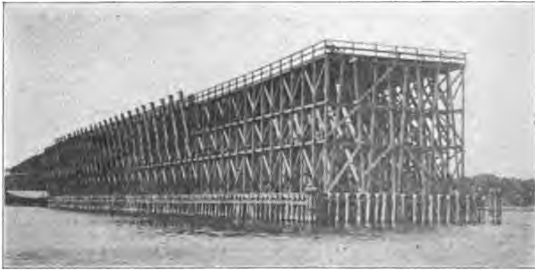
FIG. 92.—Curtis Bay pier—Baltimore & Ohio.
