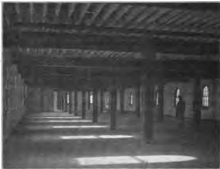
FIG. 124.—Interior of storage warehouse at Cincinnati—Baltimore & Ohio-Southwestern.
