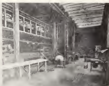
WITH CAR IN POSITION FOR INSPECTION
