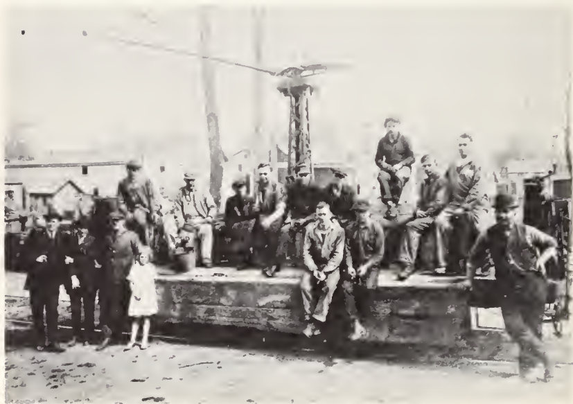
TOP - Looking east at the trolley junction about 1919 with no. 67 rounding the curve on the wye toward Brooklyn. This splendid semi-steel car was then almost new, the finest, fastest cars ever to run on the Traction being cars 63 to 73. No. 67 burned in Hempstead barn in 1923. BOTTOM - Flat no. 1 at High St. barn (Hempstead) in 1922. Larry Grella, long time Track Foreman is at extreme right
