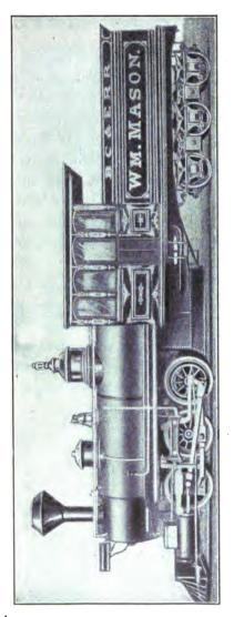
Fig. 9.-Mason Locomotive with Walschaert Valve Gear.
