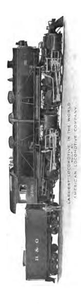
Fig. 12.—Mallet Four-Cylinder, Articulated, Compound Engine. Built by the American Locomotive Co.
