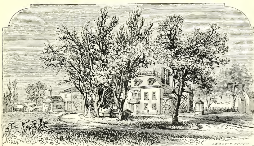
THE CORNELL-PIERREPONT MANSION. (Rear View.)
